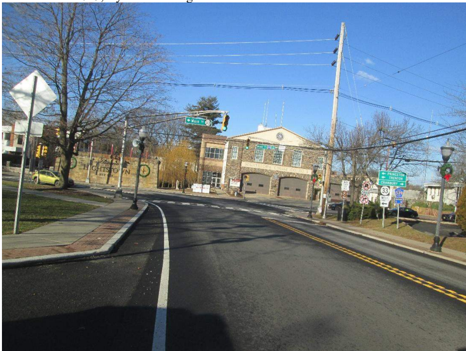
Franklin Street (Route 33) Looking West
