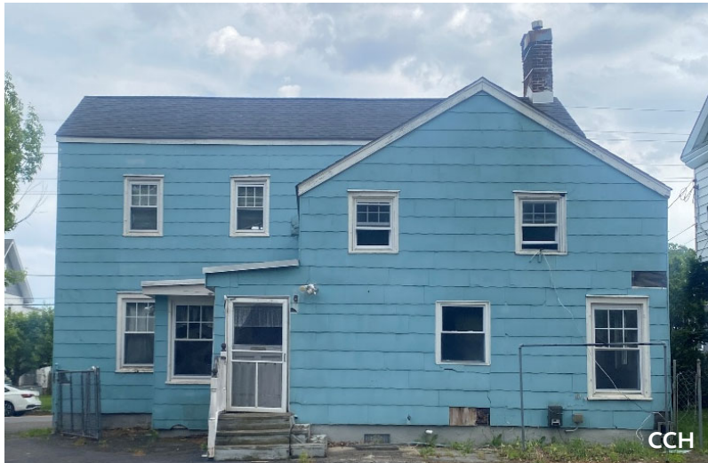
Photograph 8. Single Family House Conditions, Rear Façade.
