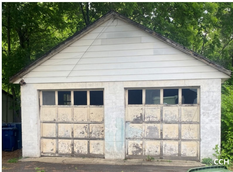
Photograph 9. Single Family House Conditions, Detached Garage.
