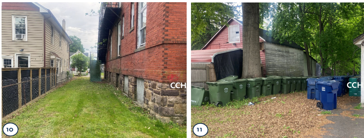
Photographs 10 and 11. Fencing to Hide View on Lot 18 Adjoining YMCA Building.
