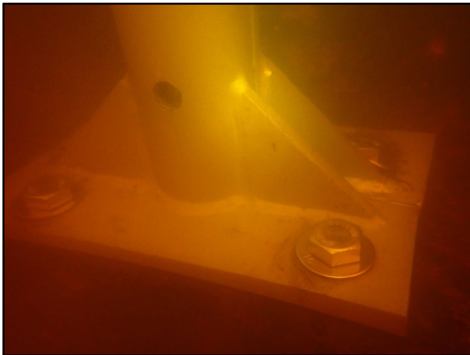
Figure 4: Riser Stem to Gate Coupler, Prior to Installing Stem Connection
