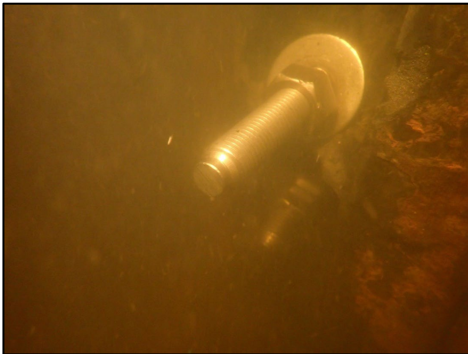
Figure 6: Double Epoxy Anchor as Installed at the Lower Left Vertical Guide
