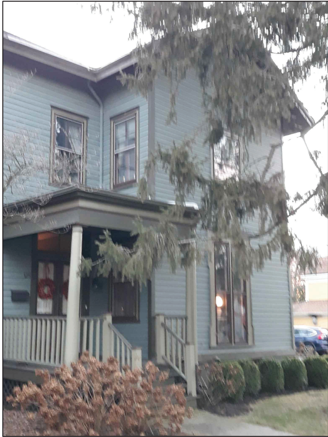
VIEW FROM SOUTH STREET
