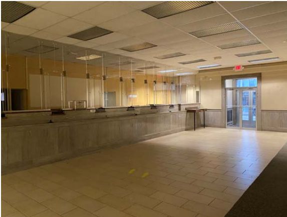
Bank Lobby with Tennessee marble and Reduced Ceiling Height
