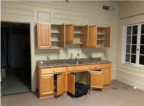
Kitchenette on Second Floor at Different Level than Addition Level
