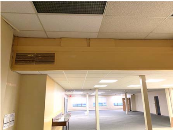
Columns Obstruct Pedestrian Flow
