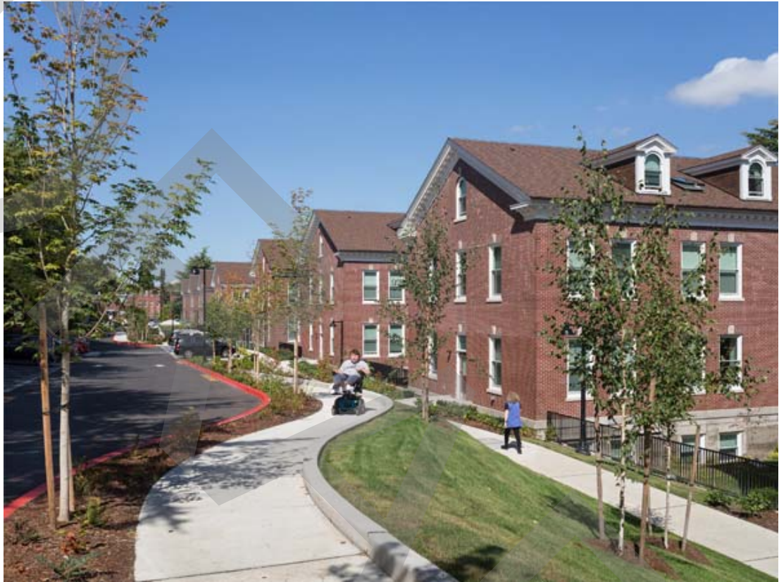
Adaptive Reuse, Affordable Housing, Seattle, WA
