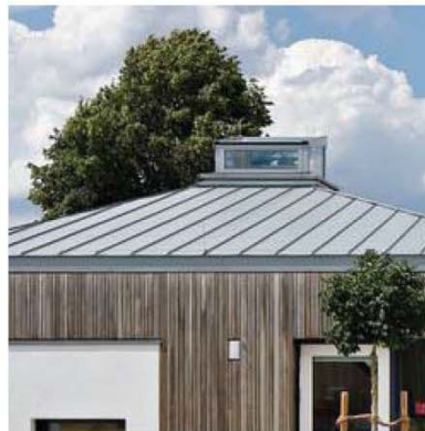
STANDING SEAM METAL ROOF Blue-Grey Finish
