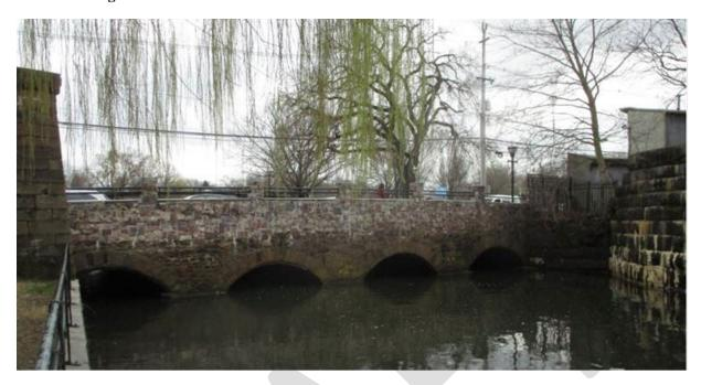
The normal water level is at the bottom of the arch. As the water level starts to rise, due to the arch shape, the opening allowing the water to flow through gets smaller and smaller. The bridge then becomes almost a dam, causing the water to build up on the lake side, eventually, flooding Main Street, the firehouse and the Borough office.
