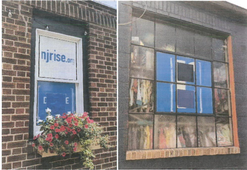
Photos of Rogers Avenue Window (left) and Parking Lot Window (right)
