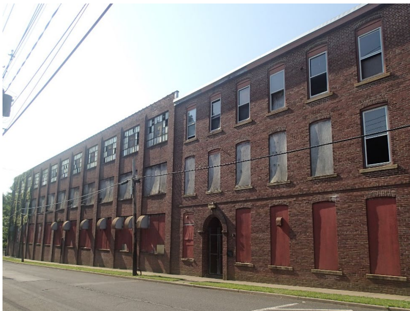
Figure 1 Brick Mill Building
