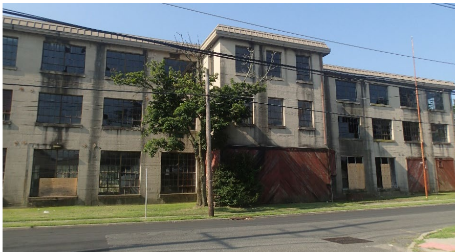
Figure 2 Concrete Mill Building
