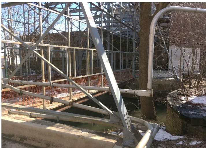
Figure 5 Footbridge over Rocky Brook
