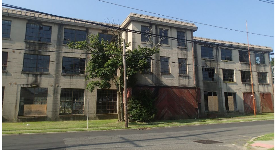
Figure 2 Concrete Mill Building
