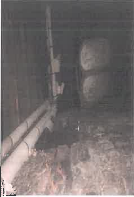
Photo 2: Basement, Old Boiler Room
