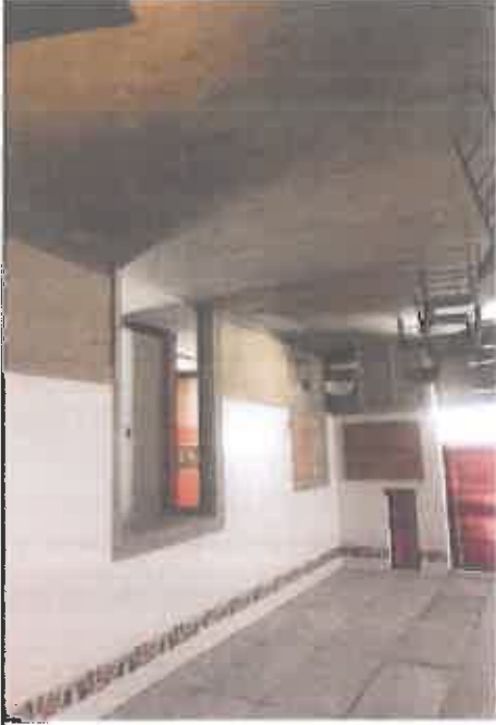
Photo 22: Ground Level, Pre School Prep Room
