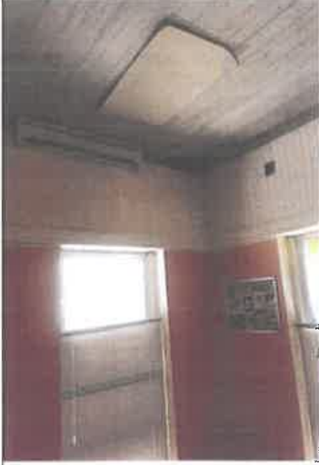
Photo 24: Ground Level, Office near Pre School Prep Room
