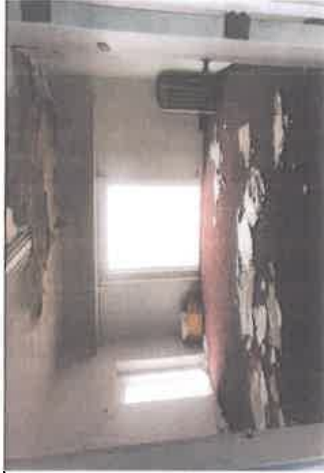
Photo 14: 2 nd Floor, Office Across Stairwell
