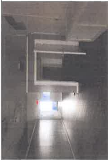
Photo 7: 2 nd Floor, Main Corridor
