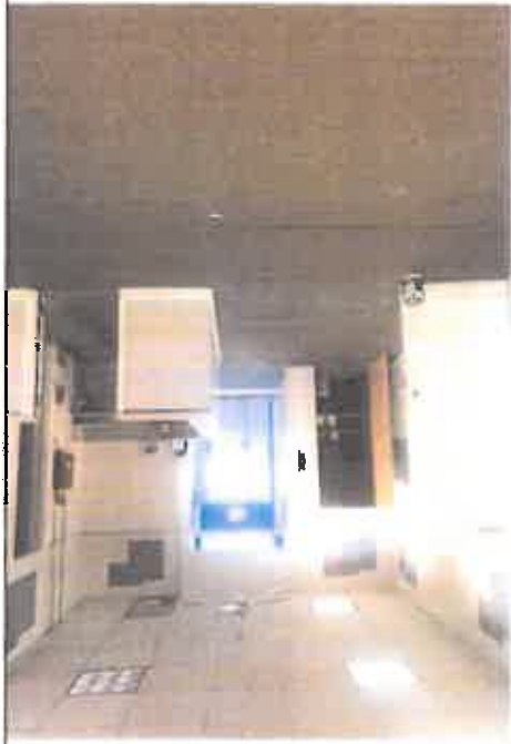
Photo 25: Ground Level, Main Corridor
