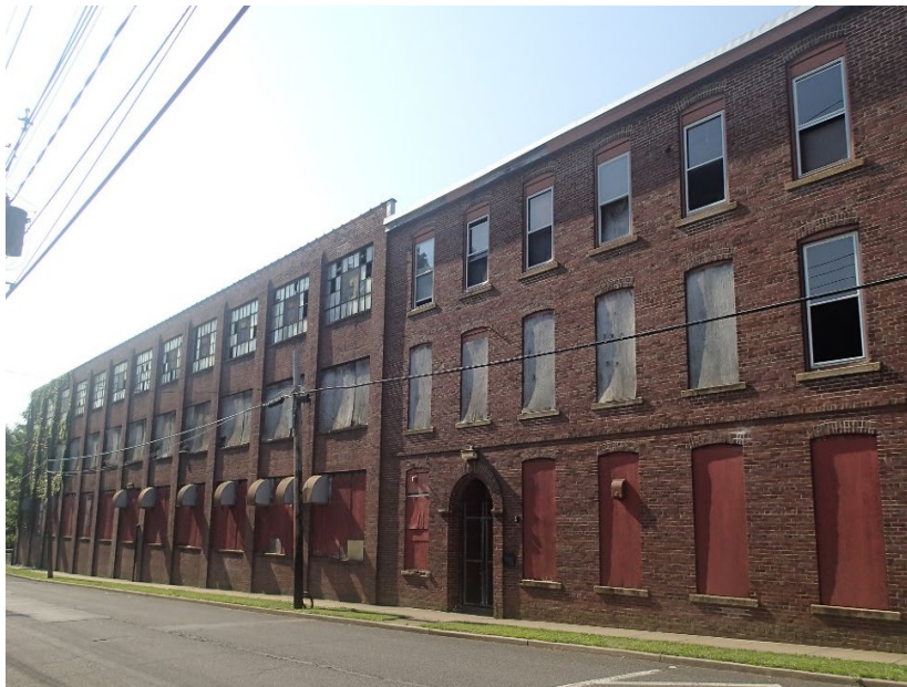
Figure 1 Brick Mill Building
