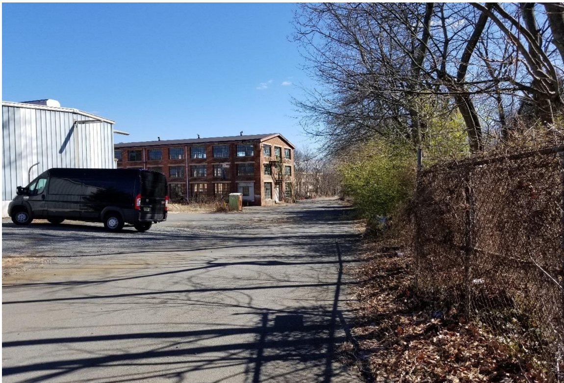
Characterizing the southwestern portion of the site and existing structures.
