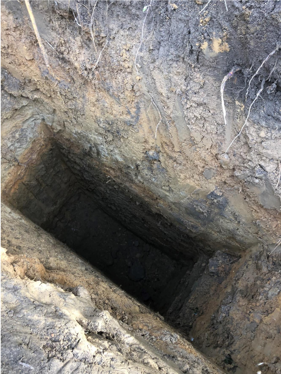
Photograph 2 – Test Pit TP-2
