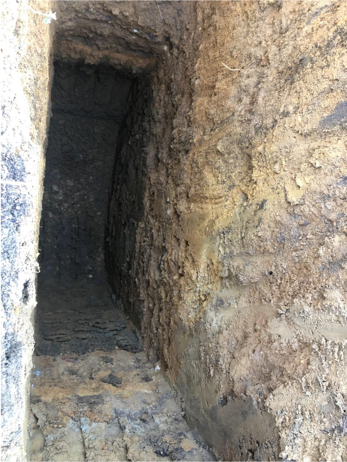
Photograph 1 – Test Pit TP-1
