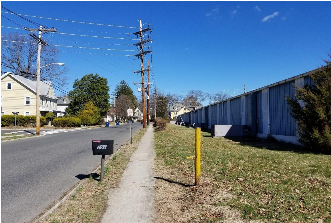
Characterizing the western portion of the site along North Academy Street and existing structures.
