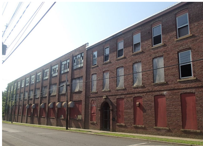
Figure 1 Brick Mill Building
