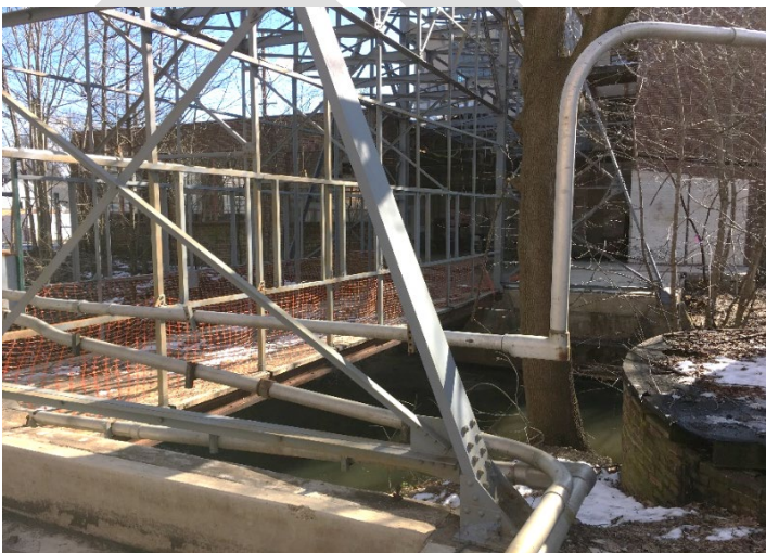
Figure 5 Footbridge over Rocky Brook
