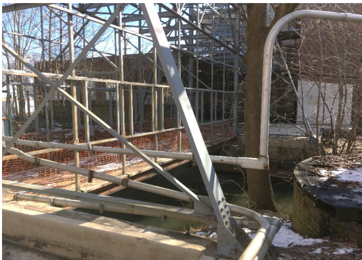
Figure 5 Footbridge over Rocky Brook
