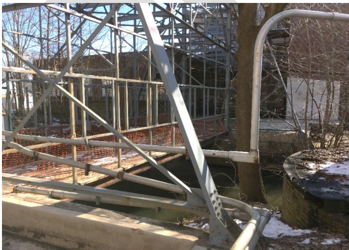
Figure 5 Footbridge over Rocky Brook
