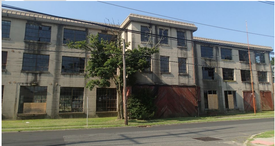
Figure 2 Concrete Mill Building
