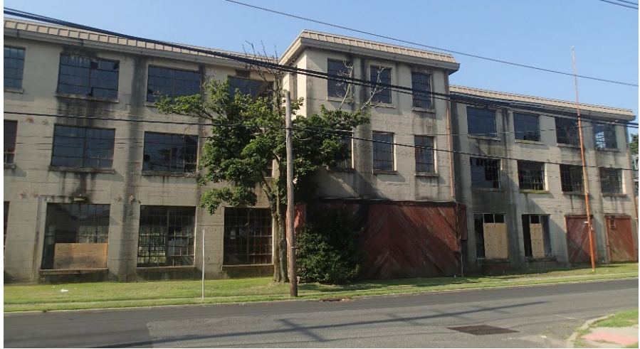
Figure 2 Concrete Mill Building
