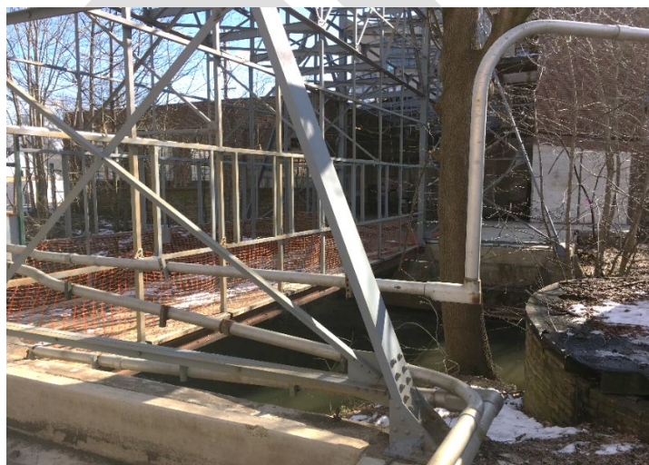
Figure 5 Footbridge over Rocky Brook
