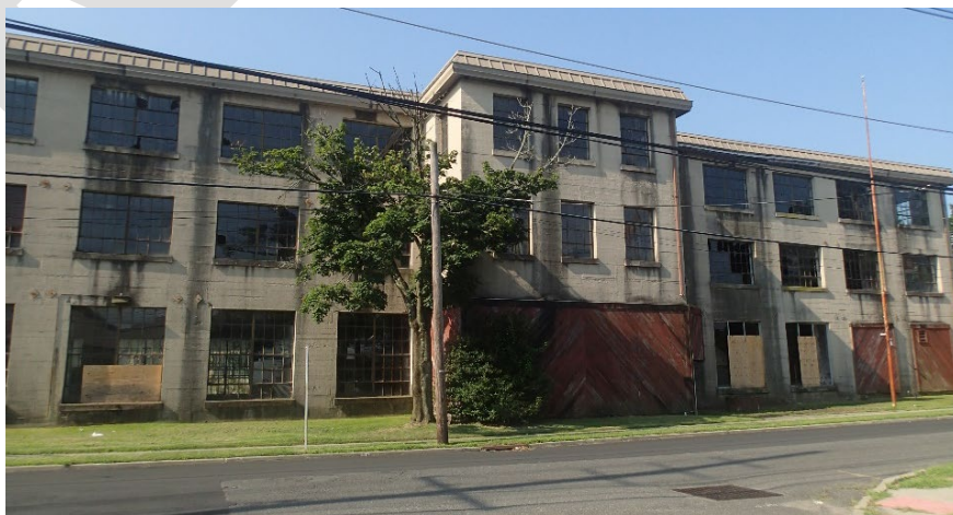
Figure 2 Concrete Mill Building
