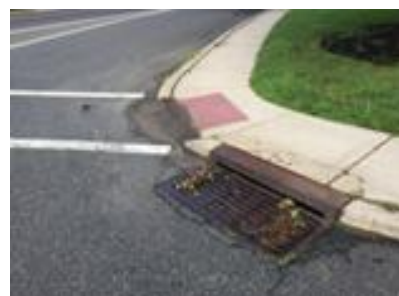
Drainage NW corner
