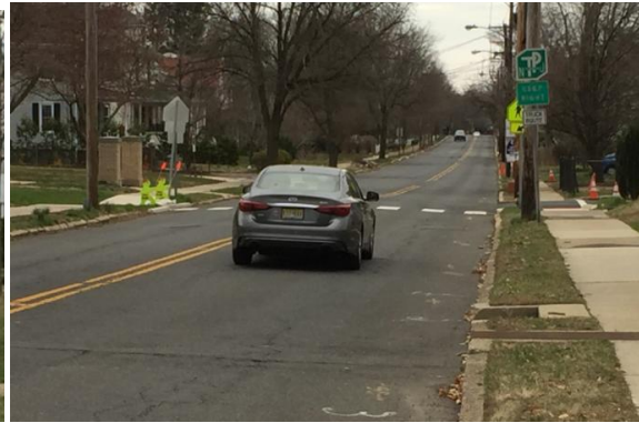
Stockton, facing east, new crosswalk
