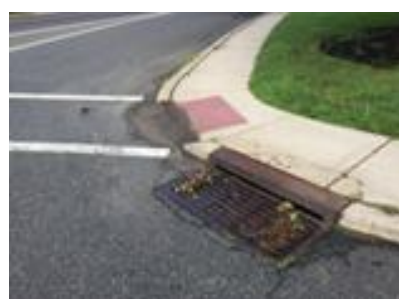
Drainage NW corner
