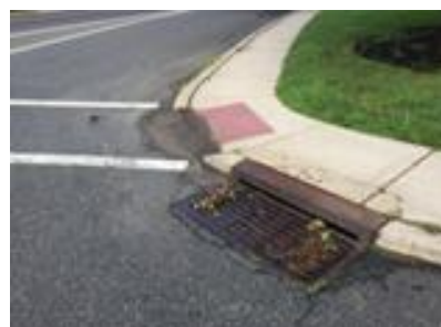
Drainage NW corner
