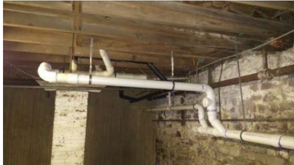
Fig. P-7 – PVC Sanitary Piping to First Floor
