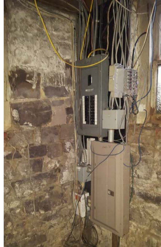
Fig. E-2- Main Service Panel A and Panel B
