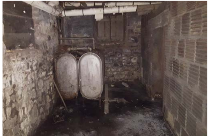
Fig. H-4- Abandoned oil tanks
