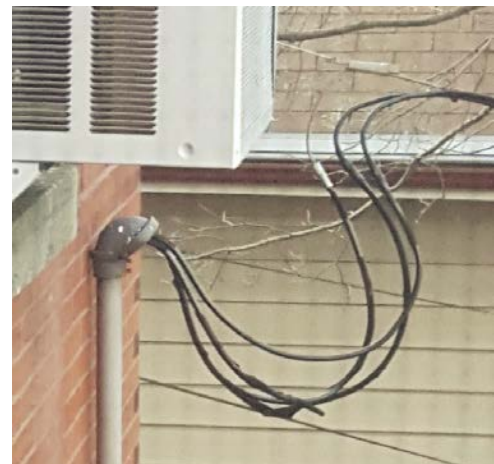
Fig. E-4- Service Wire Too Close to Window
