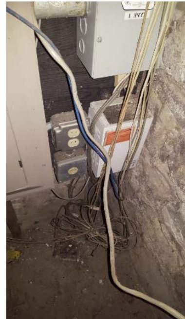
Fig. E-7- Wiring not secured per the National Electrical Code
