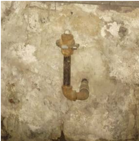
Fig. P-13- Abandoned Gas Service Entrance
