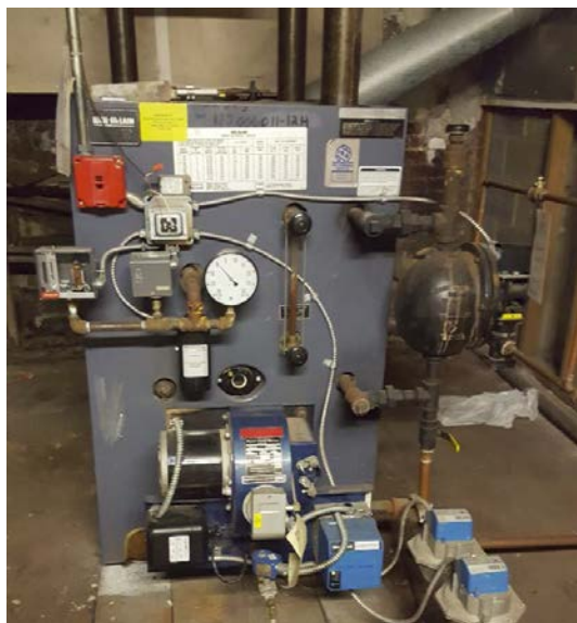
Fig. H-1- Steam Boiler
