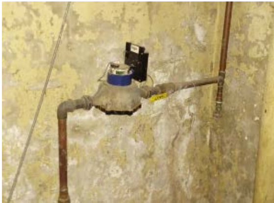
Fig. P-1-Water Meter and Pressure Reducing Valve
