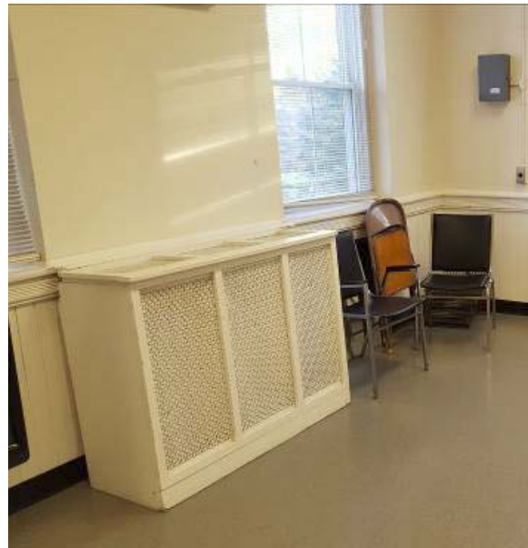
Fig. H-6- Radiator enclosure
