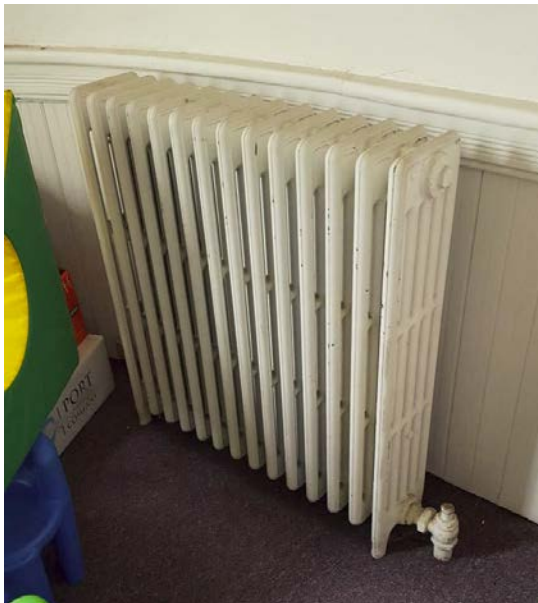
Fig. H-5- Cast iron radiator
