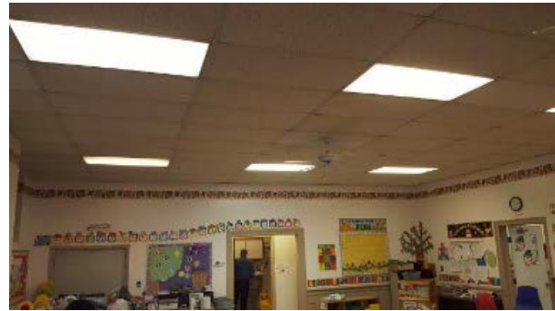
Fig. E-10- Recessed Fluorescent Lighting Fixtures
