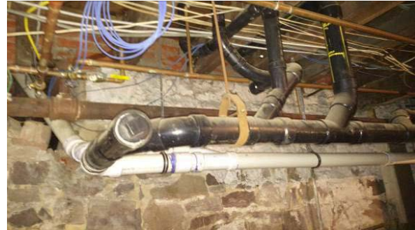
P-8- ABS Piping to First Floor
