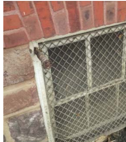
Fig. P-5- Hose Bibb (South Wall)
