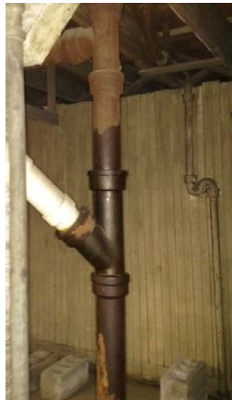
Fig. P-10- Improperly Abandoned Sanitary Piping
