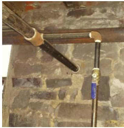
Fig. P-12 – Interior Gas Service Entrance
