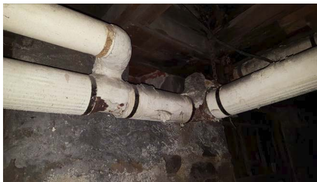
Fig. H-8- Damaged pipe insulation.
