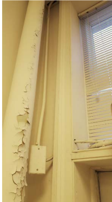
Fig. E-6- Unsecured wiring and conduit.
