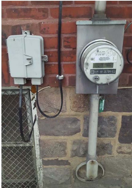
Fig. E-1- Utility Company Meter
