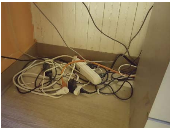
Fig. E-8- Extension cords used in place of permanent receptacles.
