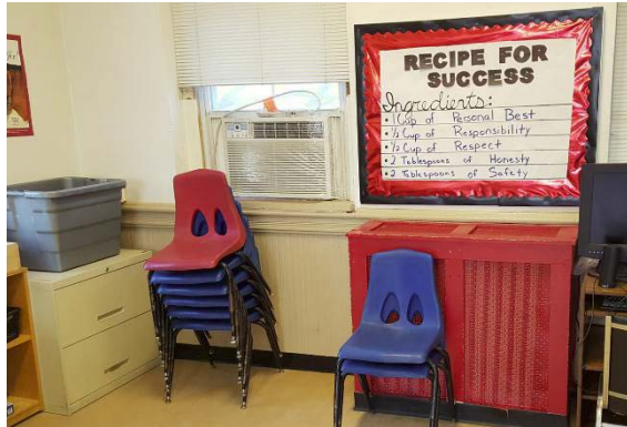
Fig. H-7- Typical window cooling unit
