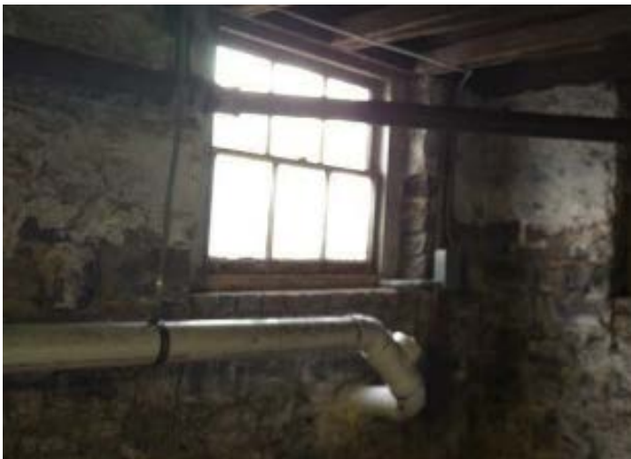
Fig. P-6 – Sanitary Sewer Service Entrance
