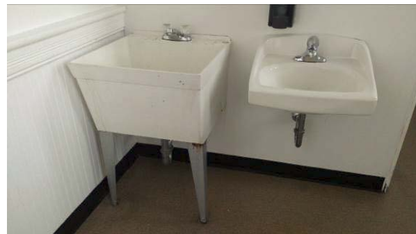
Fig. P-18 – Service Sink and Wall Mounted Sink
