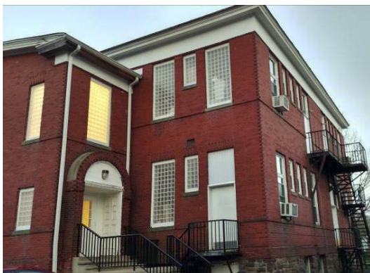
Fig. P-22- Gutters and Downspouts at Rear Entrance, The Remaining Roof Area Missing Gutters and Downspouts
