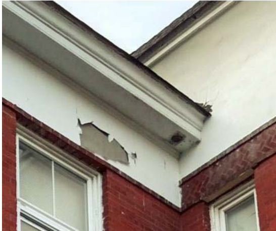
Fig. P-24- Location Where Downspout Appears to Have Been Removed
