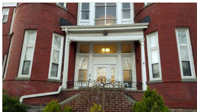
Fig. P-23- Gutters and Downspout at Front Entrance
