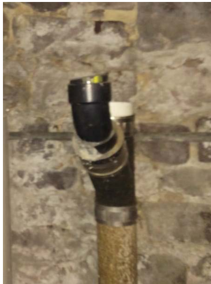
Fig. P-9- Improperly Abandoned Sanitary Piping
