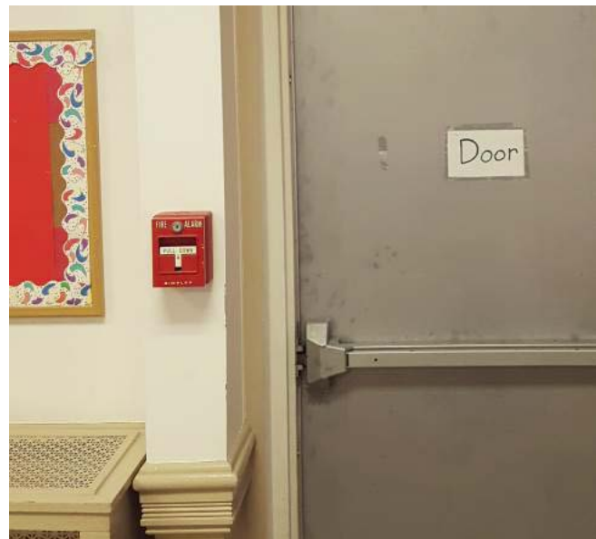
Fig. E-15- Fire Alarm Pull Station
