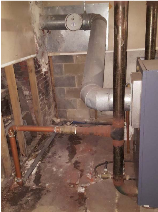
Fig. H-3- Boiler flue to chimney
