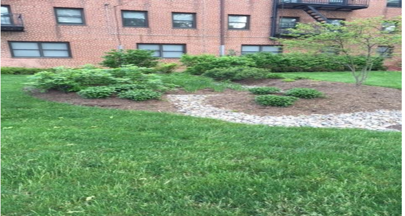
Building 2 Rain Garden
