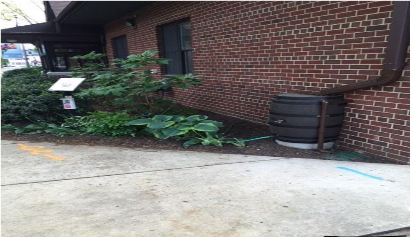
Rain Barrels with percolating trenches
