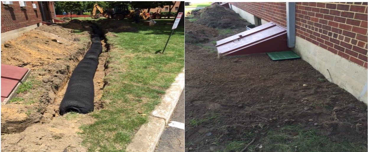
Installation of pervious lateral trenches to distribute storm water runoff into the soil.
